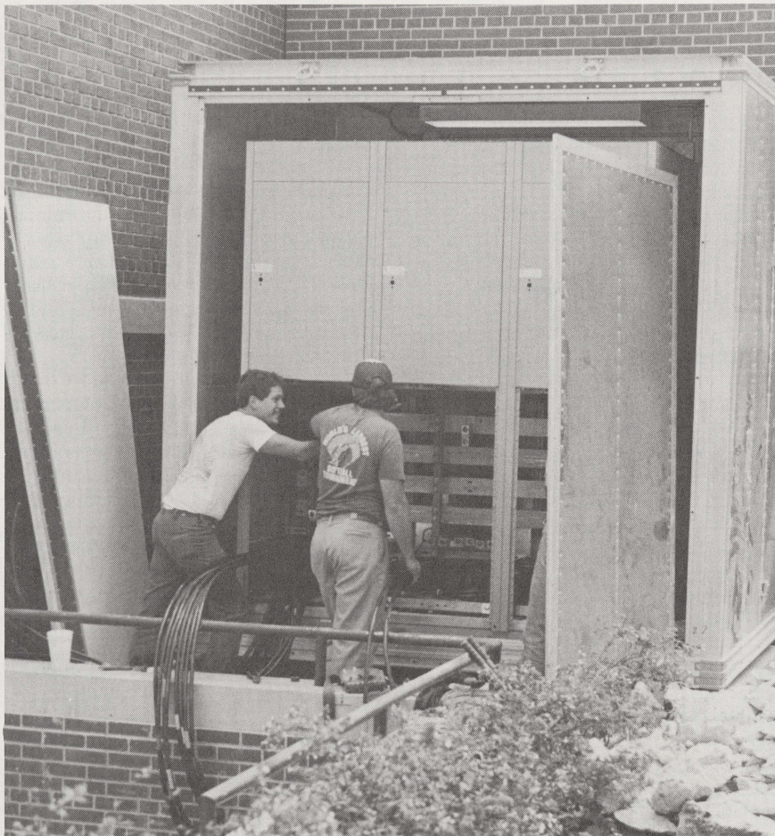
No, it's not an oversized trunk or a big freezer. Workers install parts of the synchronizing switching gear for two backup generators that supply emergency power for EMG and several nearby buildings.
