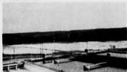
There are 2 sludge (waste) lagoons behind the water treatment plant. Waste from the plant is held here.
