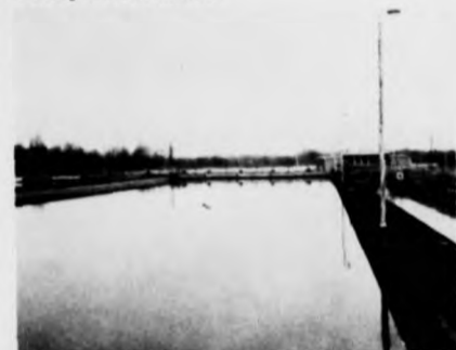
This is one of eight sedimentation basins at the Morse Road water treatment plant. They are 350 feet long and 70 feet wide each! Six hold 4 million gallons of water and two hold 4,600,000 gallons of water.
