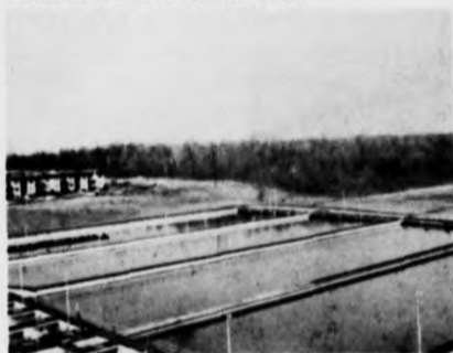
Here are four of the eight sedimentation basins at the water treatment plant. This picture was taken by Cheryl Prusinski from the roof of the 5 story building.
