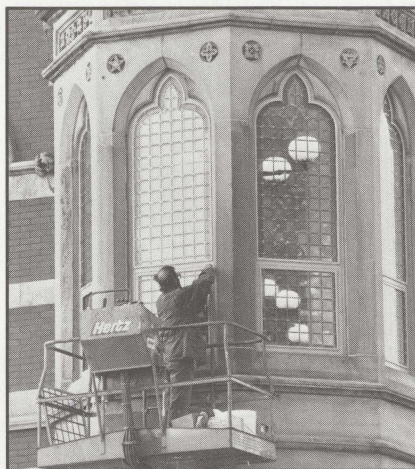
(LEFT) A workman adds historically accurate leaded glass exterior windows to the President's Office in College Hall. (RIGHT) A stone mason cuts out a block of Chapel Hall's original sandstone face to replace it with a new block.
