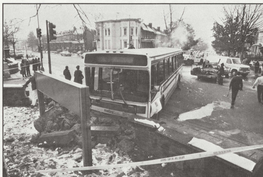
A Metrobus heavily damaged a section of Gallaudet's 100-year-old sandstone wall on Florida Avenue near the Eighth Street entrance Feb. 14 after a collision between the bus and a car. A passenger in the car died and about six people sustained injuries.
