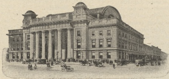
Chicago Passenger Terminal, Chicago & Northwestern Railway.
